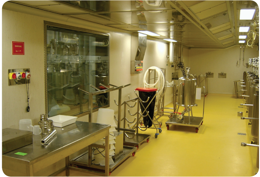
Clean room: cold storage room at -5^{\circ}\text{C} classified in class C.
