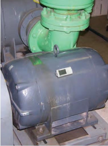
HOBO UX90-004 Motor On/Off data logger records motor on/off status.
